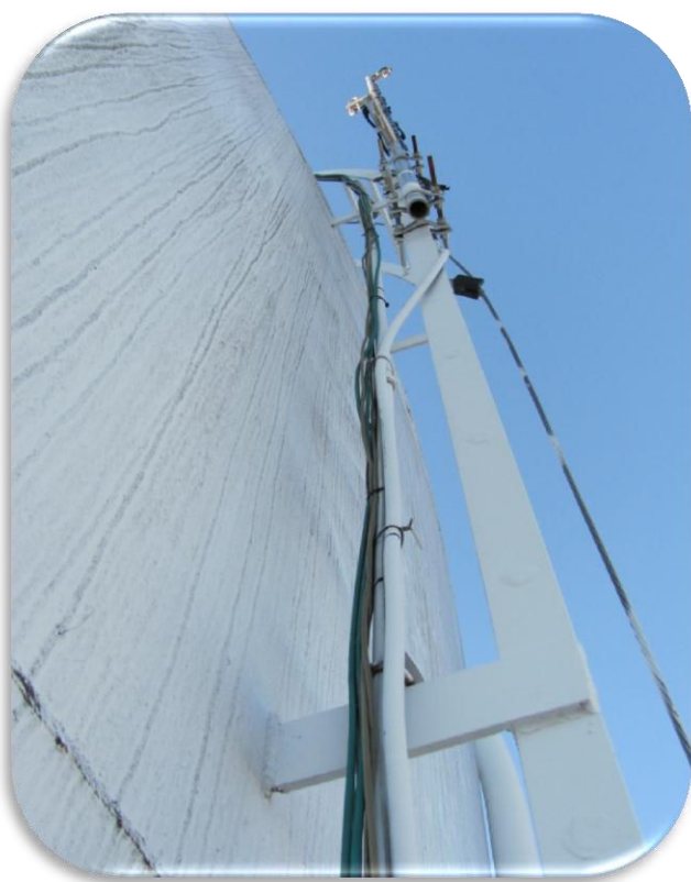
Photo 2 (access ladder with violating cable/conduit on stand-off bracket)
