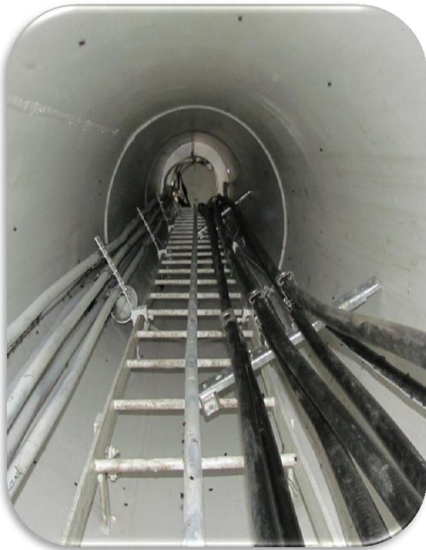
Photo 1 (a cellular company has installed cables on the side and face of ladder)
